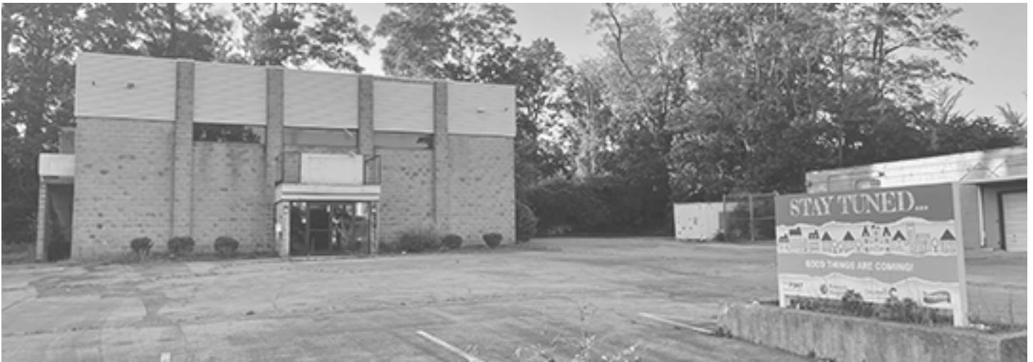
The old Spotlight property at 6543 Montgomery Rd. will be the future home to affordable senior housing.
