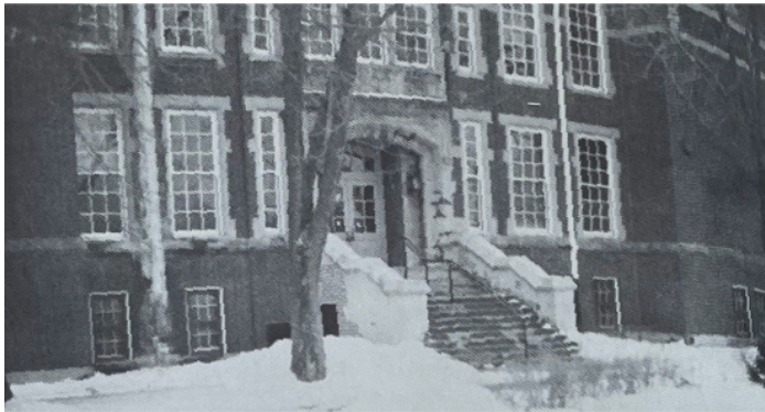
Kennedy Elementary School, built in 1912
