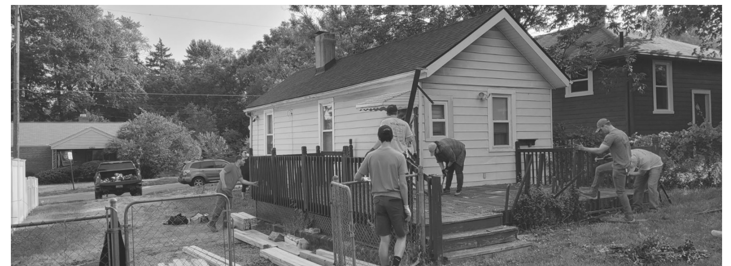
Volunteers helping in the new Home Repair Program.
